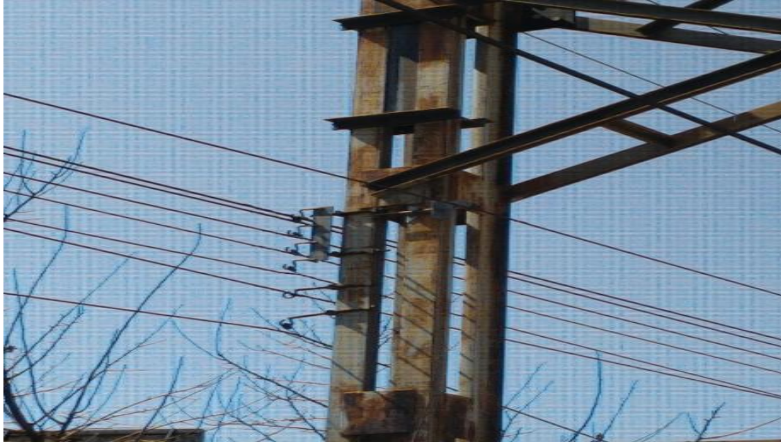
Figure 1.3.1 OPTIC FIBRE AERIAL WITH SUSPENSION BRACKETS
